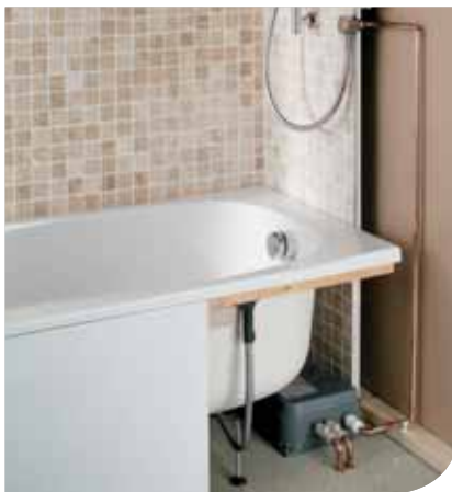
Under bath installation - use otherwise un-used space behind the bath panel
